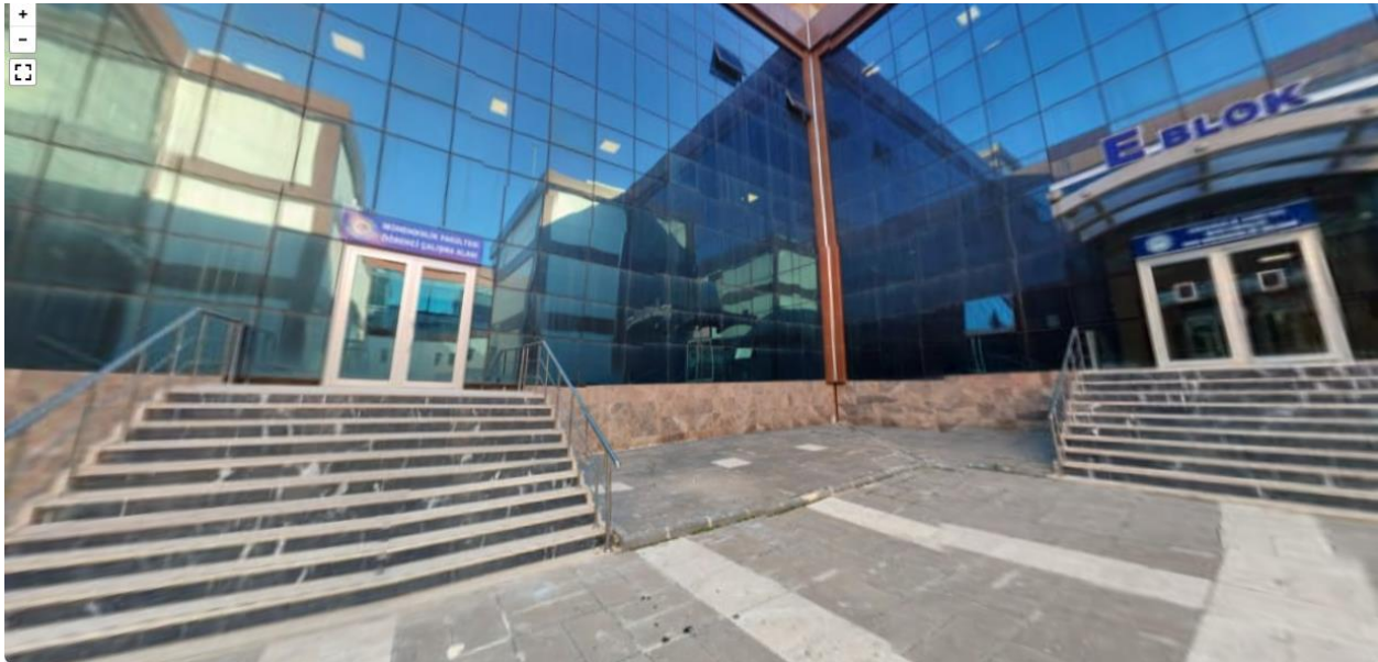
Figure 4a. Building: Engineering Faculty
