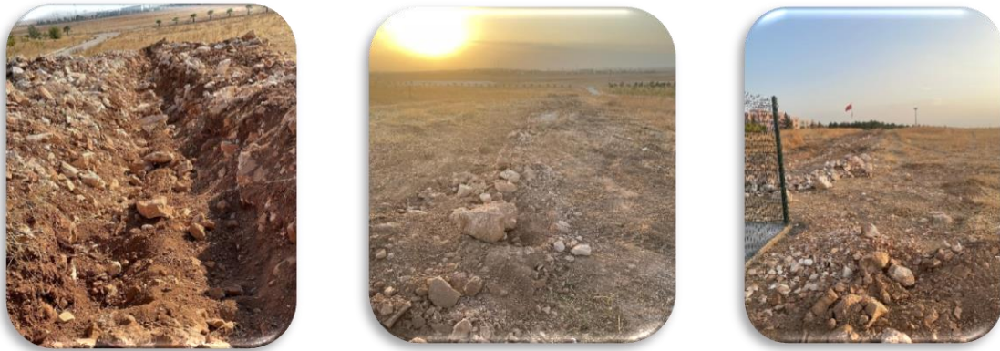
Figure 8. Covering Trenches with Rocks and Soil
