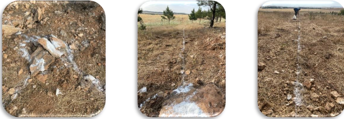
Figure 3. Ground Marking for the Lines
